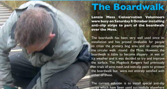
The current solution is to install special anti-slip strips which have been used successfully elsewhere and this is now a project in progress. Feedback so far has been very positive.
